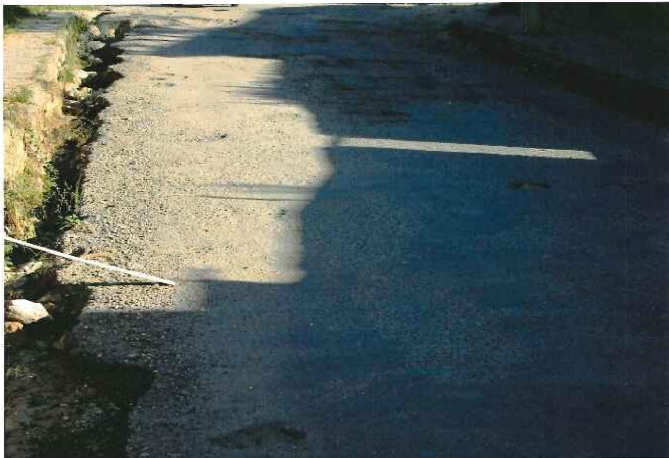
FIGURA 136 – VIAS COM GRANDES BURACOS DEVIDO A FALTA DO SISTEMA DE DRENAGEM.
